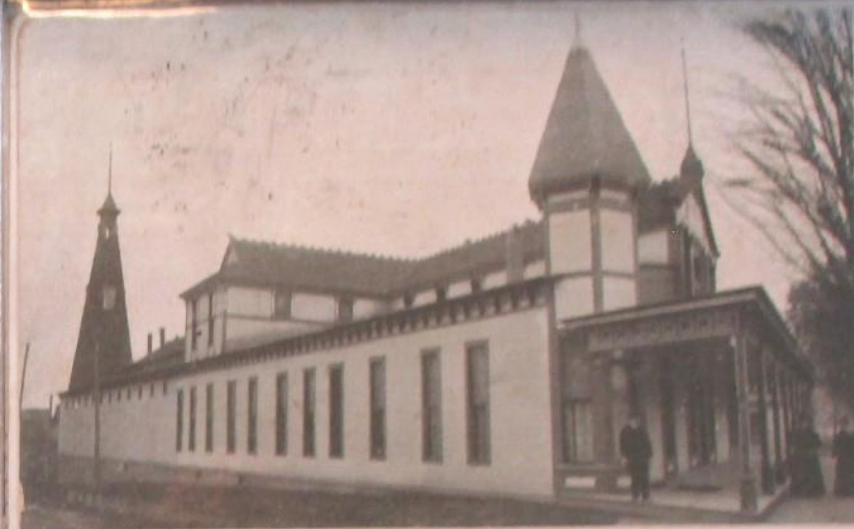
FOUNTAIN BATH HOUSE, MT. CLEMENS, MICH.
